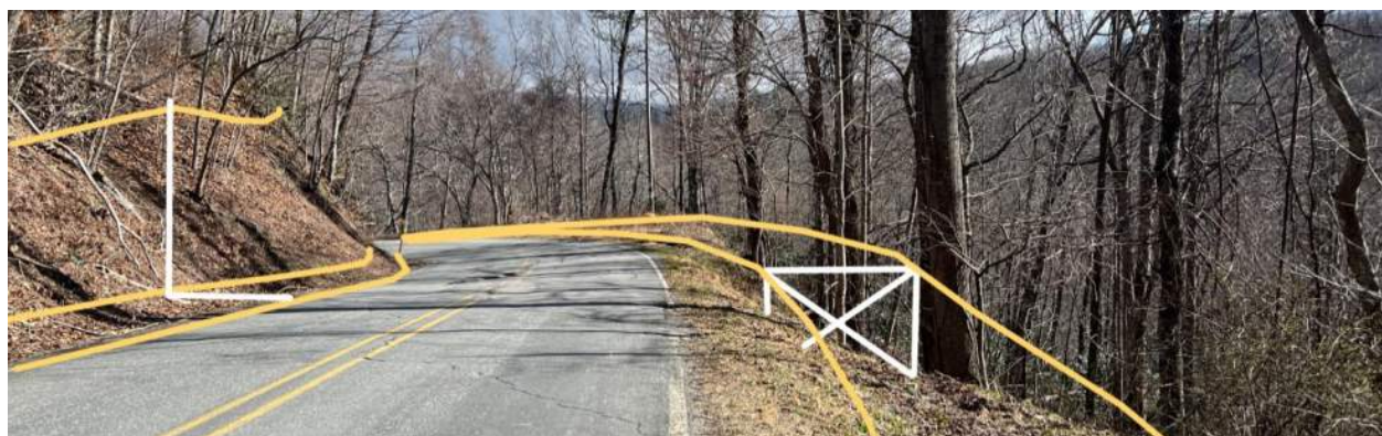
Figure 48. Diagram of Mill Creek Rd. Options – Segment D1 upslope trail alignment with cut and retaining wall structures (left) vs. Segment D2 downslope trail alignment with modular boardwalk (right)
